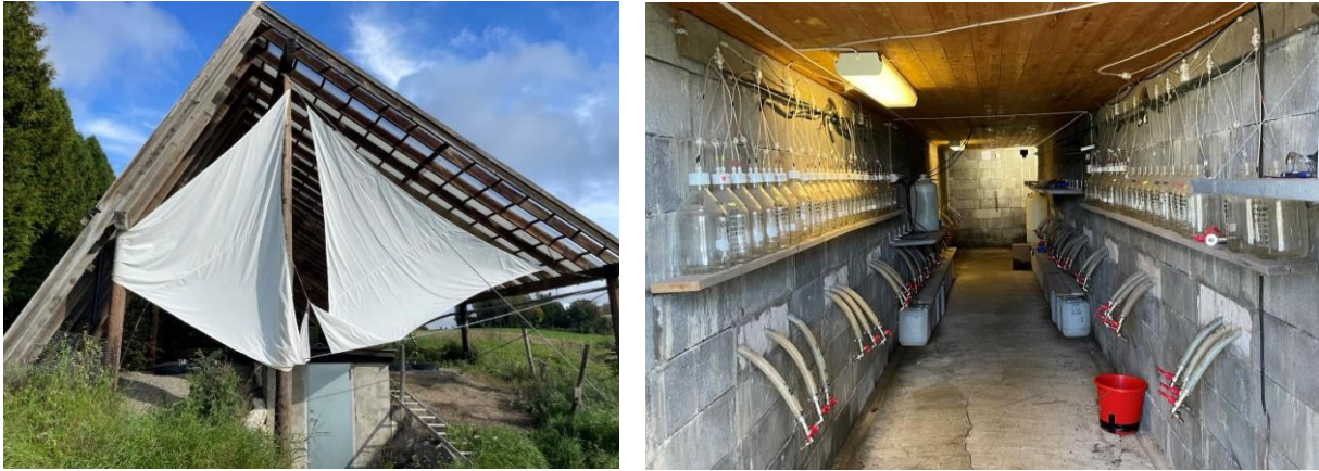
Figure 4: Facility improvements included installation of white sails to prevent direct sunlight through the front opening (left), and mounting of stop cocks on the outlet pipes in the cellar for drainage management (right).
