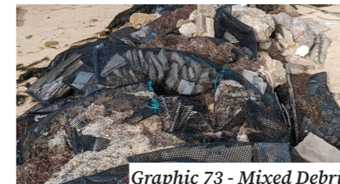
Graphic 73 - Mixed Debris Piled together or collected in mesh bags, the material are used to reduce erosion.
