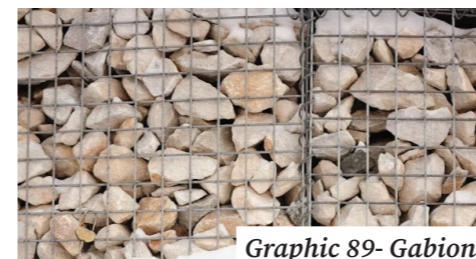
Graphic 89- Gabions Walls, as boundaries or erosion control, can be cheaply erected in gabion cages.
