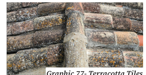
Graphic 77- Terracotta Tiles More traditional roof material. Have also been used as decorative garden elements in Faro.
