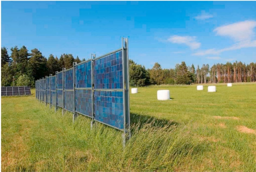
Figure 12. Campana et al. (2021). Bifacial photovoltaic modules in a vertically mounted agrivoltaic system at Kärbo Prästgård, Västerås, Sweden. Optimisation of vertically mounted agrivoltaic systems . Journal of Cleaner Production , 325, p.18 s. https://doi.org/10.1016/j.jclepro.2021.12909
