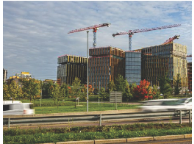
Figur 7: Construction City i Hovinbyen. Foto: Construction City.
