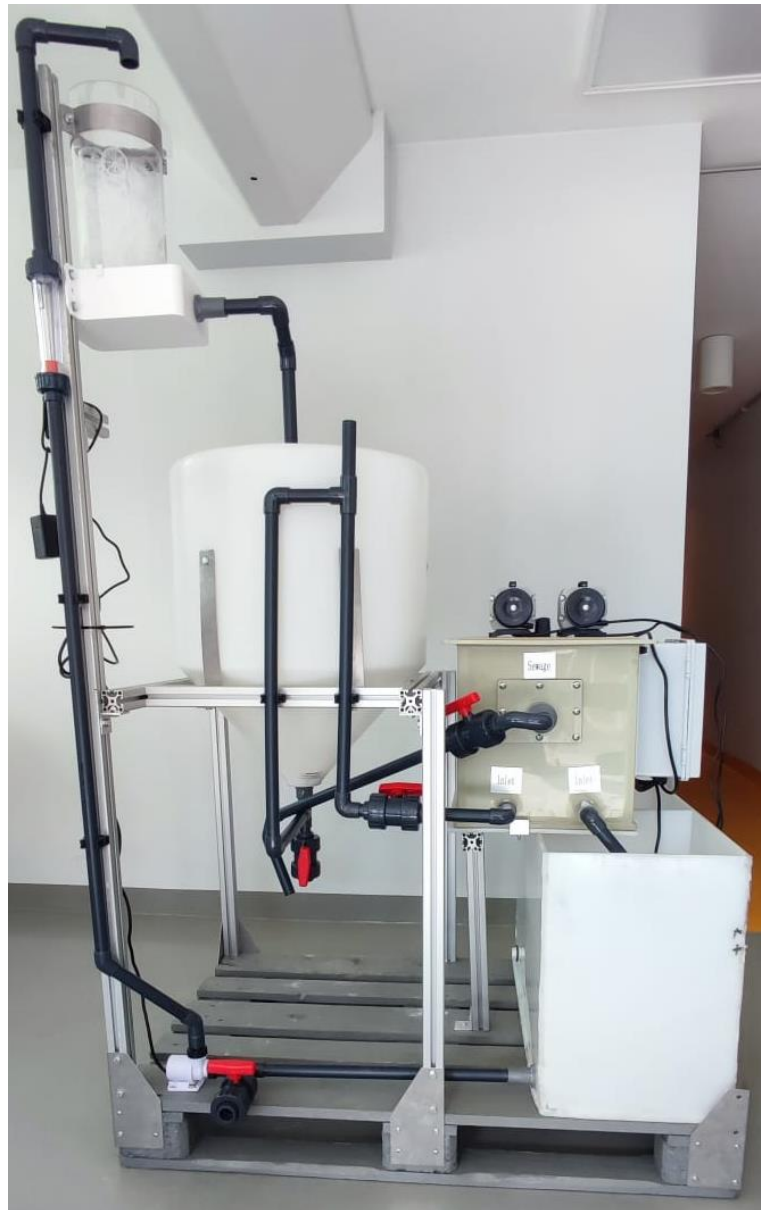
Figure 5. 1: The right-side view of the finished RAS unit
