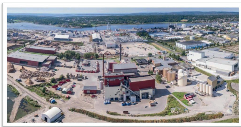
Figure 10. FREVAR KF biogas facility (FREVAR KF 2018).
