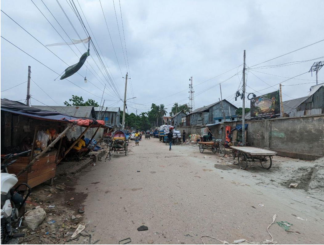
Fig.26: Concrete wall on both sides of Adeal Road to separate the Korail Slum
