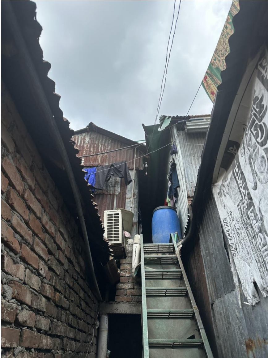
Fig. 53: Narrow stairs of a typical two-storied house in Korail.
