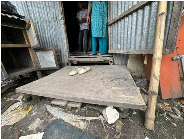
Fig. 54: The house is elevated to stand against flooding of Lake
