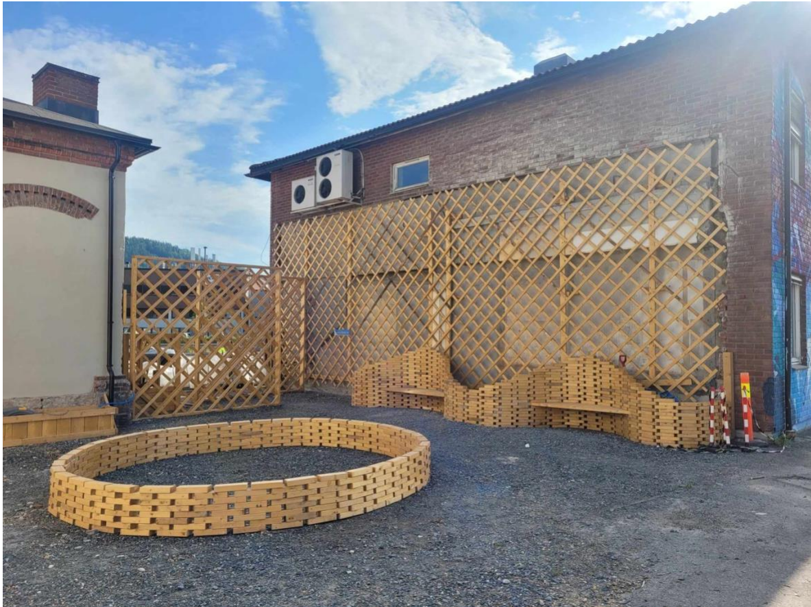
Figure 33 Sustainable use of cuts off from plank at Godsden constructed by students from Åssiden High School based on ideas from Omtre
