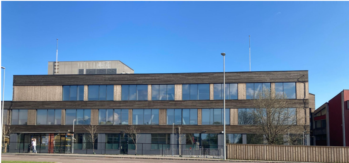
Figure 3.2: Picture of Ås High School (orientation corresponds to spans seen in the BIM-model for different levels)
