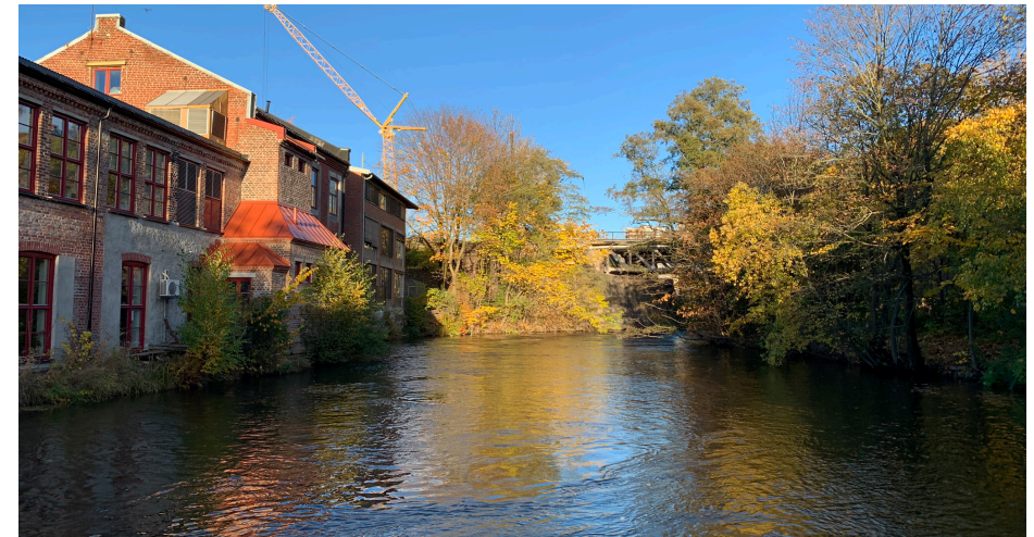
Fig. 38 View of the upper basin, as seen from the dam.
