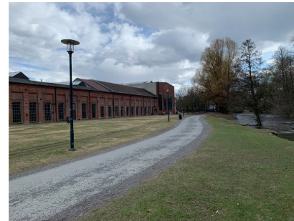
Fig. 34: The main pathway and the eastern industrial facade, south-eastern perspective
