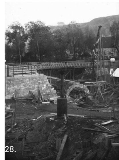
Figure 28: Working on closing the Alna River by the hospital.
