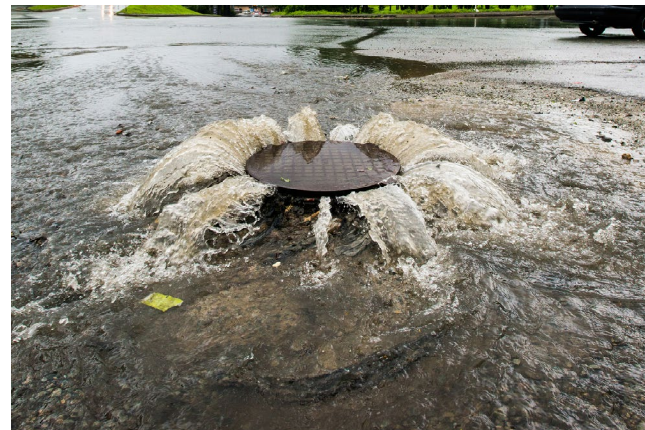
Figure 7: shows an example of a piped drainage overflowing Source: watercolor managment, n.d.
