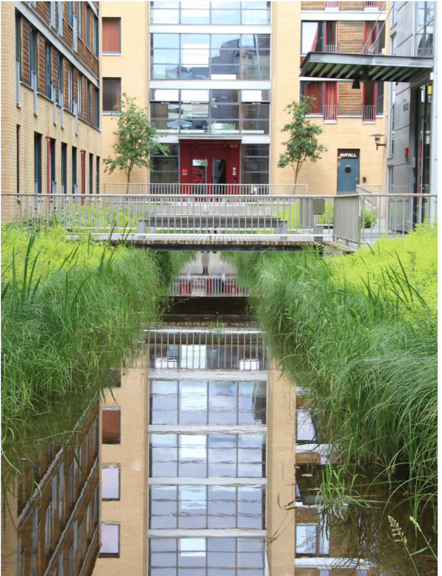
Figure 3: Bjølsen student city, an open stormwater canal between the residential blocks (Miljødirektoratet, 2022)
