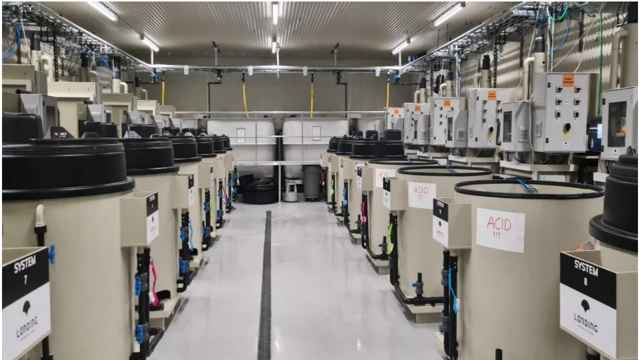
Figure.4 Single RAS system: NOFIMA, Sunndalsøra
