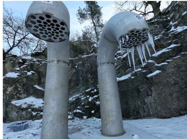
(c) View from below of the goose neck gratings which are 400 mm in diameter.
