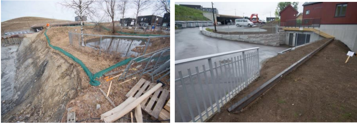
Figure 3. The left picture is Kjeller dam gård during development from 2013 to 2016, plastic guiding fences have been put up to guide the animals along a safe path to and from the pond. The right picture is the back of the building facing Kjeller gård pond, the pond is straight ahead. The metal is the guiding fences for the animals, and the wooden path along the building is the newt bridge, which lead the animals away from the road to the left. Pictures were taken by Jeroen van der Kooij.
