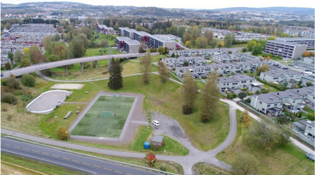
Figure 2.2 Photo of Bråtenveien towards Glostrupdumpa and onwards to the north, taken with a drone by Multiconsult (2019) Retrieved from: (Multiconsult, 2019), figure 4 drone photo of Glostrupdumpa, photo: Multiconsult
