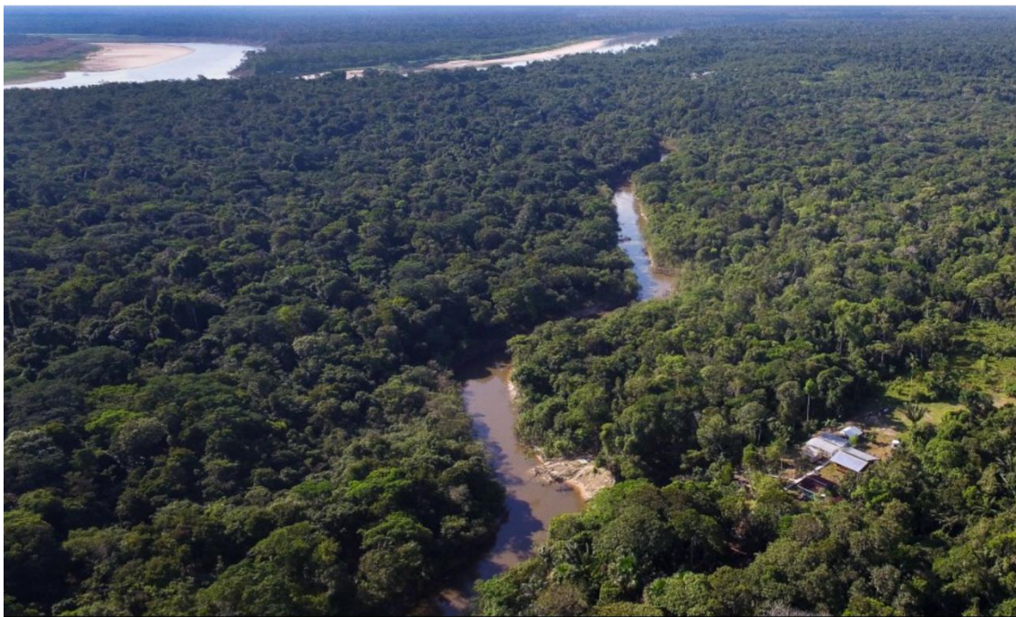
Figure 13: Aerial image of the Forest Products Processing Unit at Bauana community, with the Juruá River in the background.
