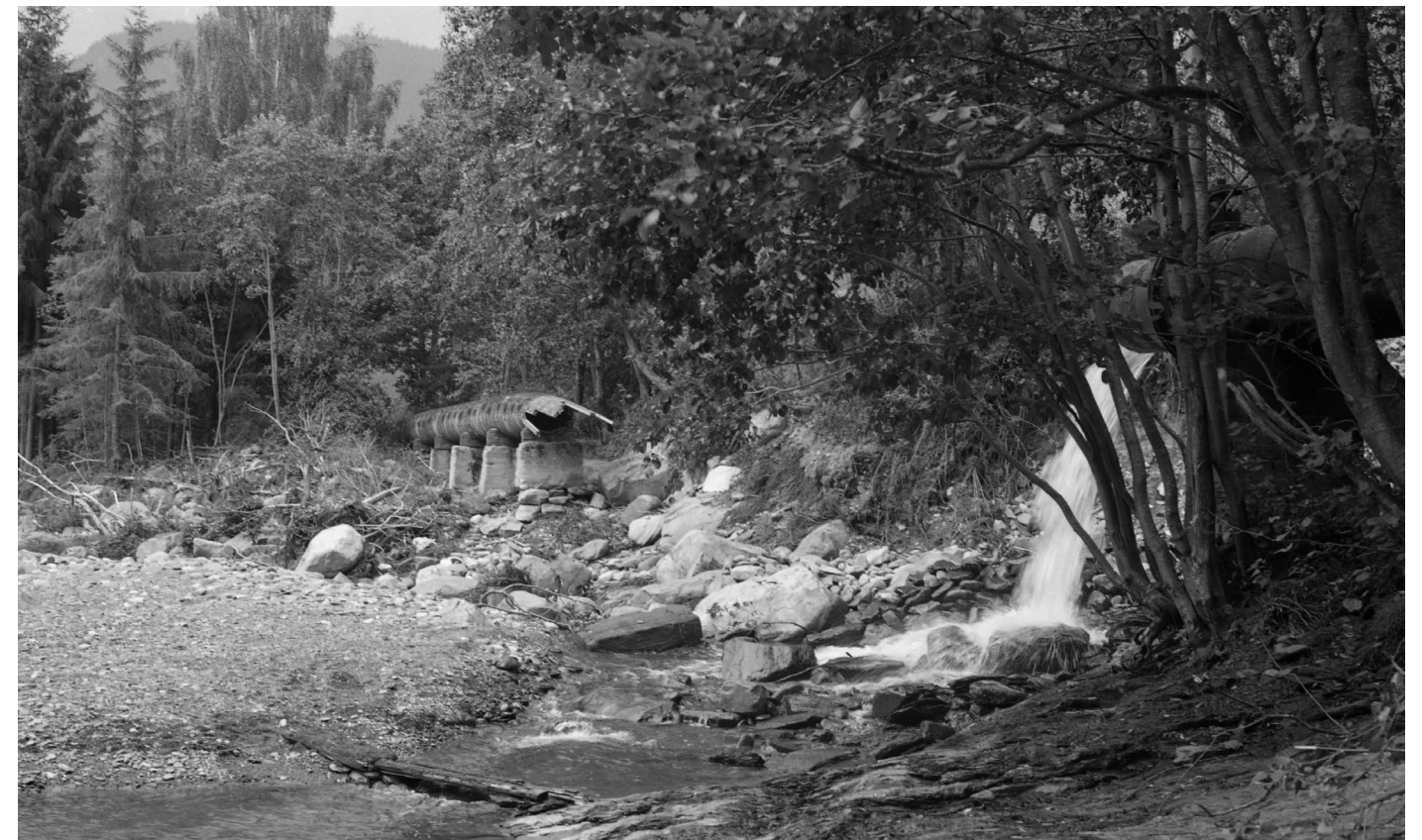
Figure 9b: A spring flood broke the pipes of the dam at Tromsa river, in 1985 (Photo: Sparby, K., 1985).
