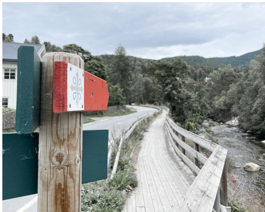
Figure 60b: Extended pedestrian walkway along Tromsa towards the dam site and the High bridge (Photo: Fjeldberg, I. 2022).
