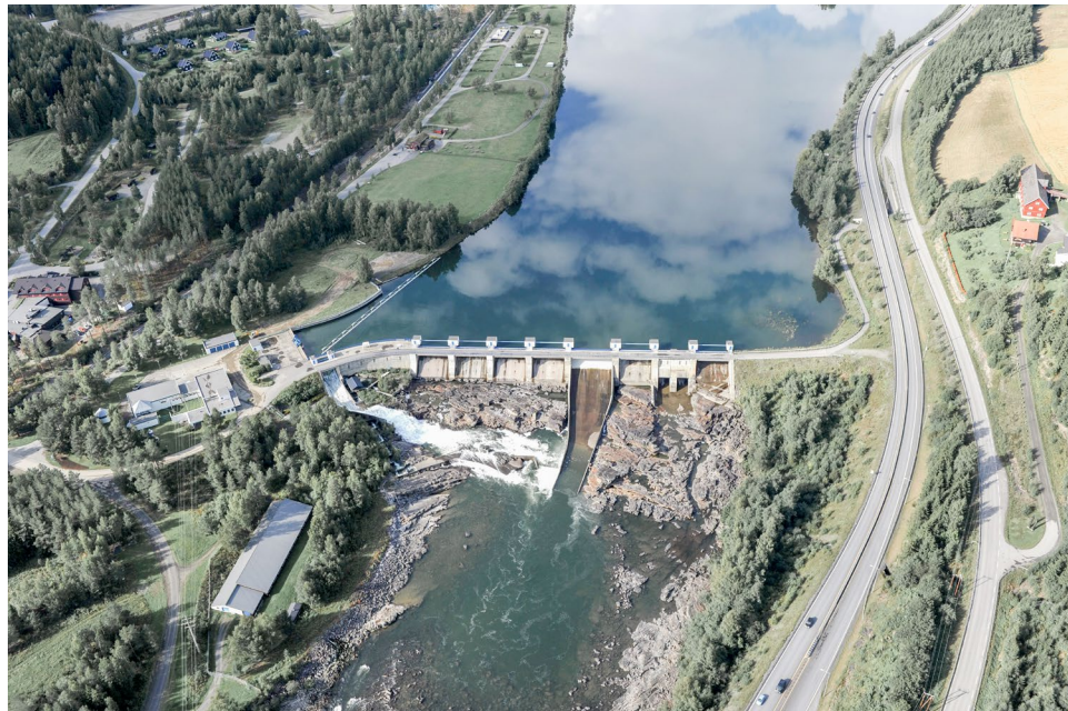
Figure 21b: Hunderfossen hydropower dam (Photo: Hafslund Eco Vannkraft).
