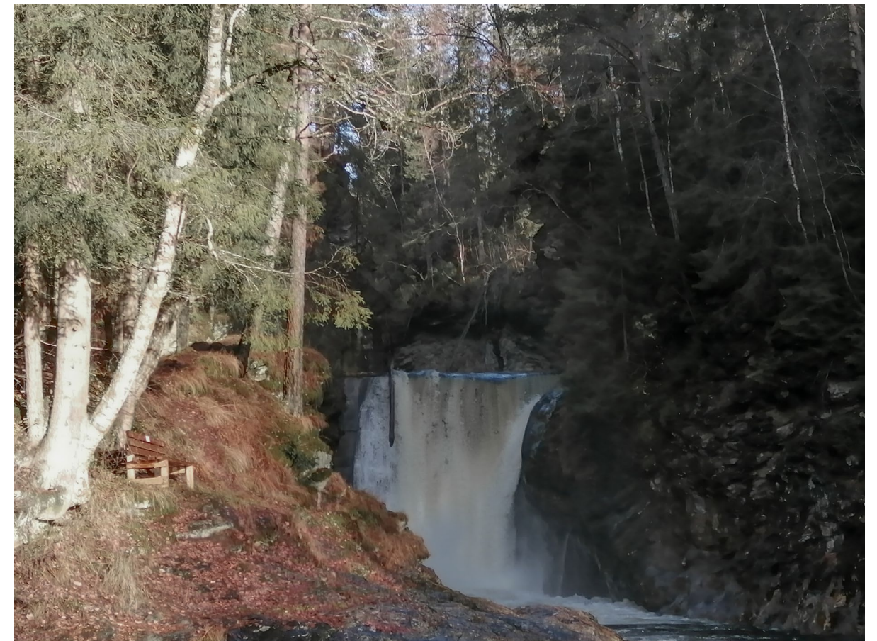
Figure 45c: Closer view of the dam before removal (Photo: Ringlund, O. 2020).
