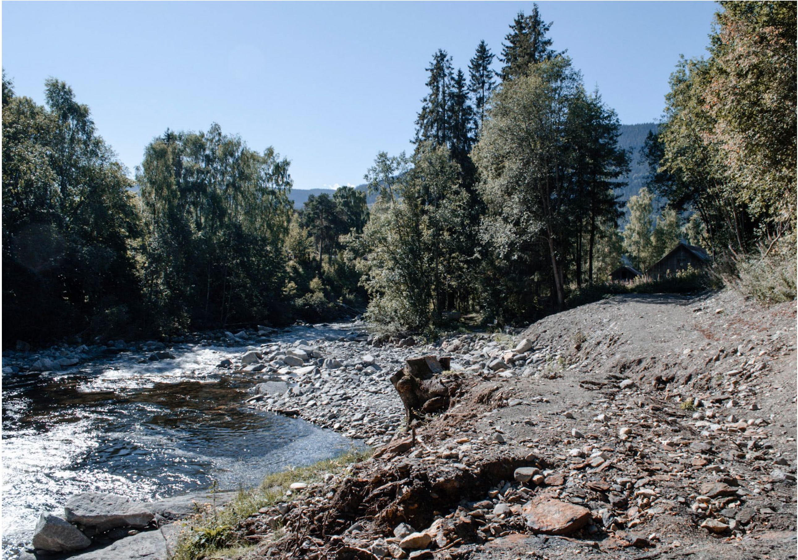
Figure 59e: View of Tromsa, with the temporarily constructed road that was washed away by the spring flood on the right (Photo: Fjeldberg, I. 2022).
