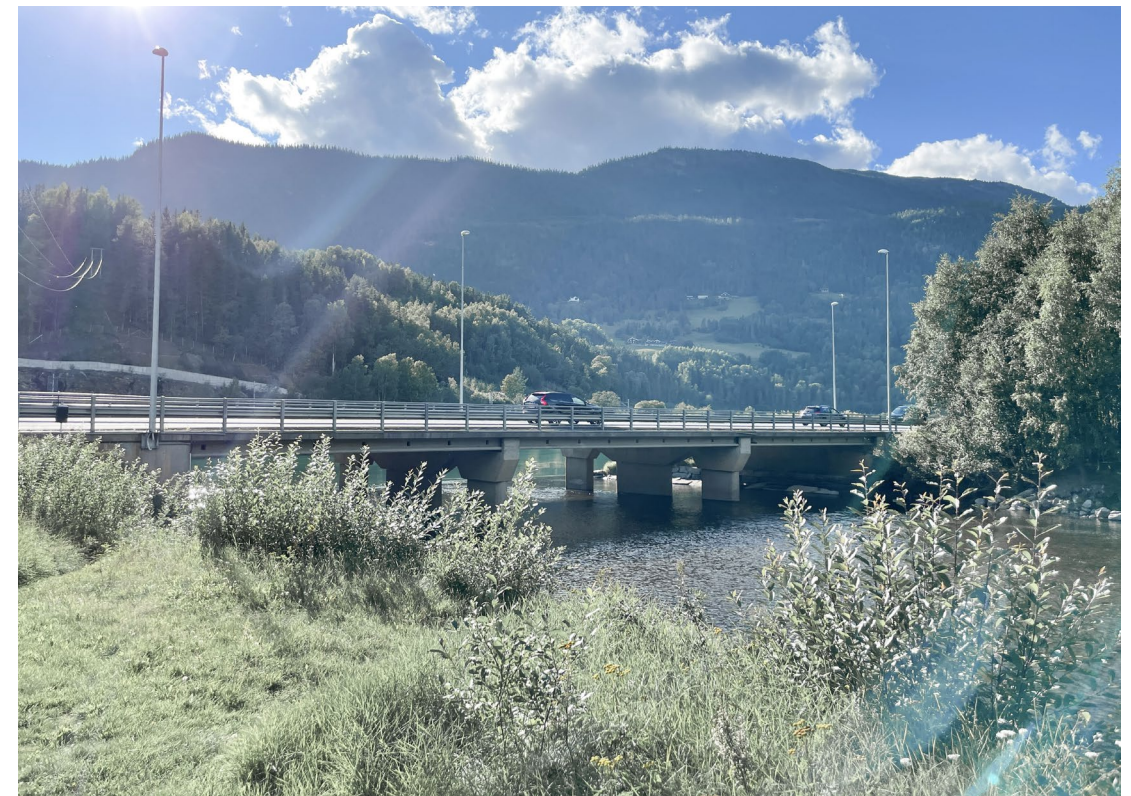
Figure 62f: Highway E6 at the outlet of Tromsa (Photo: Fjeldberg, I.).
