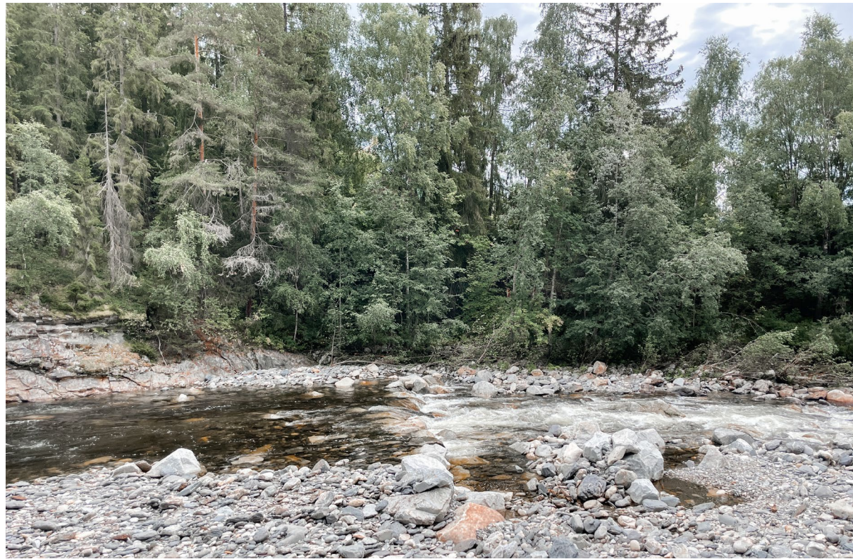
Figure 21d: Thresholds constructed in the Tromsa river after the removal of the dam (Photo: Fjeldberg, I. 2022).
