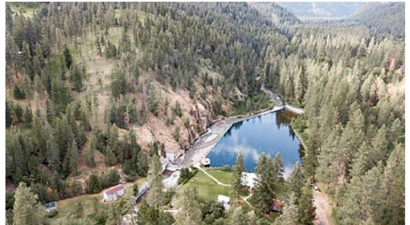
Figure 16c: The site before removal of the dam (Image source: City of Missoula, 2018).
