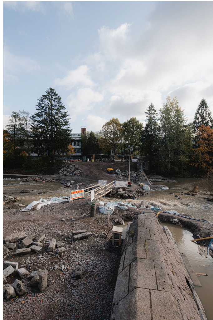
Figure 13: Removal of the Tikkurila dam in Finland (Photo: Pyry Kantonen Photography, 2019).
