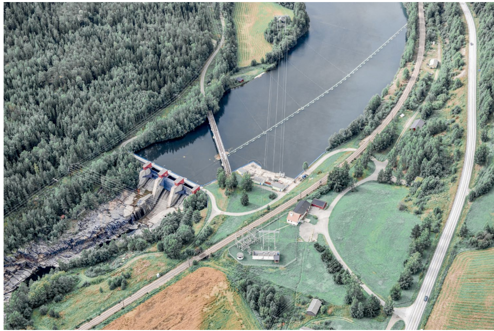
Figure 21a: Harpefoss hydropower dam (Photo: Hafslund Eco Vannkraft).
