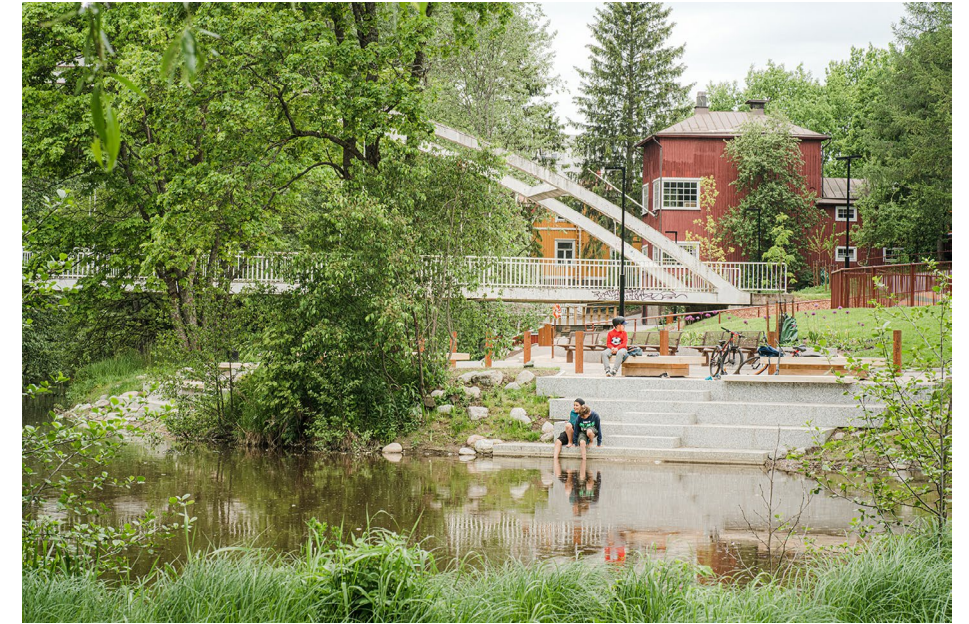
Figure 15f: Parts of the dam is preserved and included in the design as a cultural monument (Photo: Pyy Kantonen Photography, 2019).
