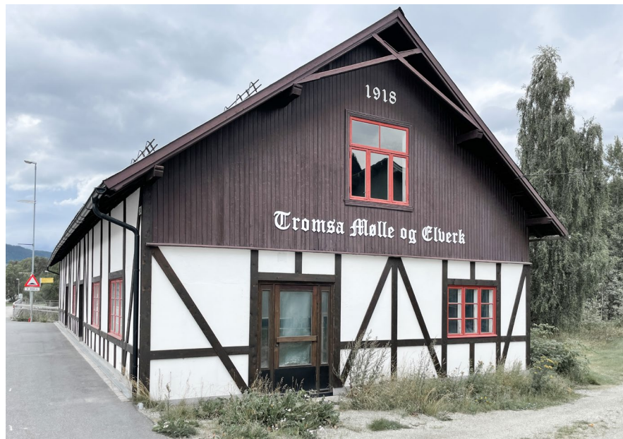
Figure 44a: Hydropower was produced in the basement of this building (Photo: Fjeldberg, I. 2022).
