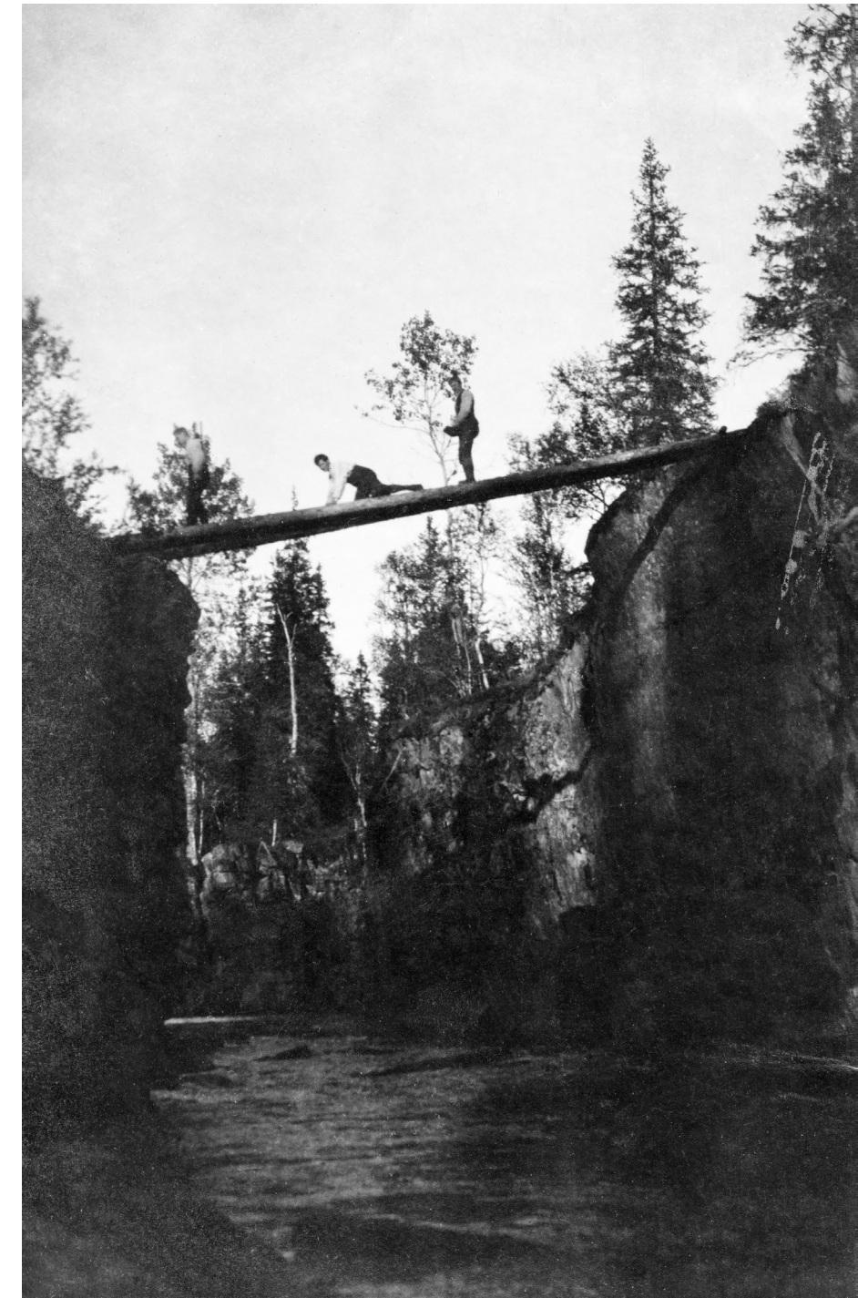
Figure 42c: "Dangerous passing over Tromsa at Trones" (Vigerudst, A. no date).
