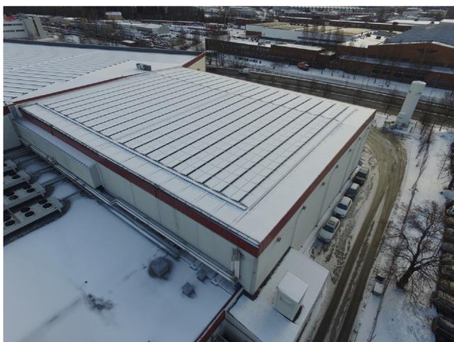
Fig. 1. A PV snow mitigation system installed on a warehouse in Oslo. The system is designed by Innos [12].
