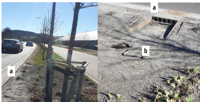
Figure 1. Left picture: the bioretention cell is the area located between the road and the sidewalk. Right picture: inlets specially designed and fitted to the side curb bring road runoff to the bioretention cell. A 13 cm high side curb (a) separates the road from the bioretention cell. Sampling spot in front of an inlet (b).
