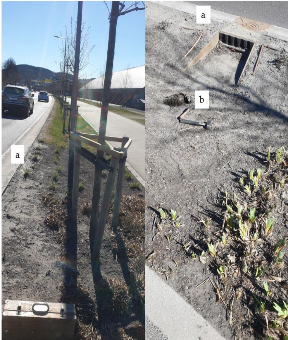
Figure 6. Left picture: bioretention cell located between the road and sidewalk . Right picture: inlets specially designed and fitted to the side curb bring road runoff to the bioretention cell. (a) A 13 cm high side curb separates the road from the bioretention cell, (b) sampling spot in front of an inlet.
