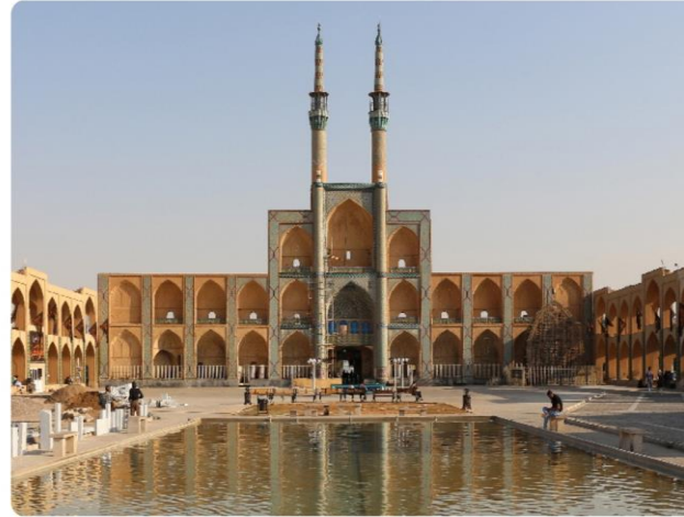
Figure 57: Amir Chakhmaq Complex
