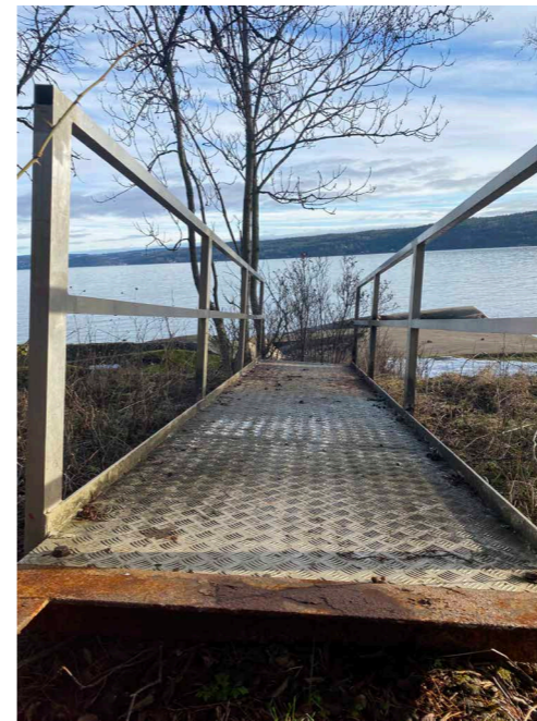
Handicapped ramp for water access
