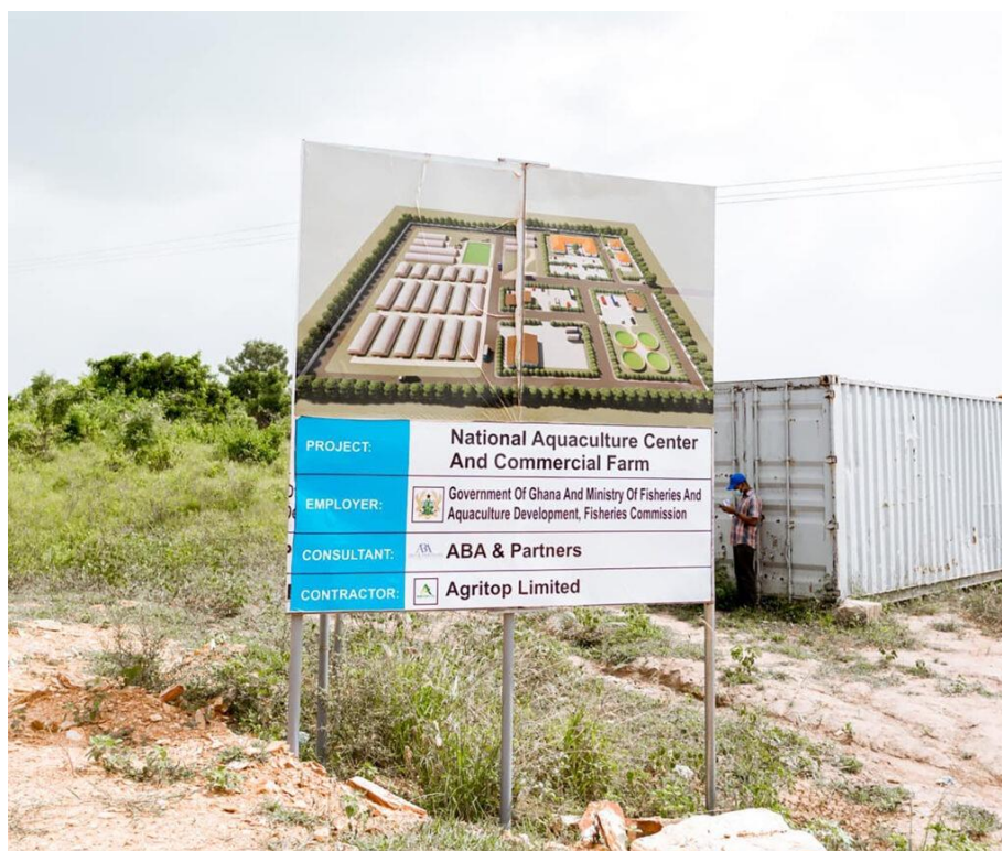
Image 9: Site plan of the new National Aquaculture Center And Commercial Farm in Amrahia, Ghana. Photo credit: Aquaculture magazine, Source: (Magazine, 2022)
