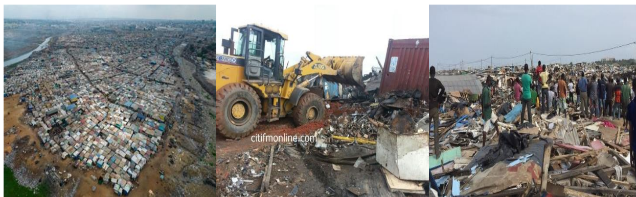
Figure 3 Old Fadama Before, During, and After the Demolition Exercise
