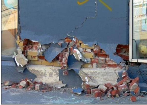
Figur 25 - Kantknusing (toe-crushing) (Dizhur et al., 2011).
