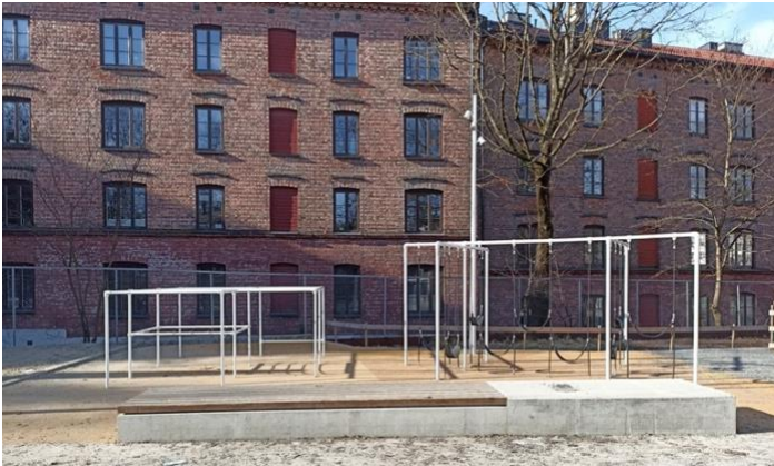
Figure 13. Picture of zone 7
