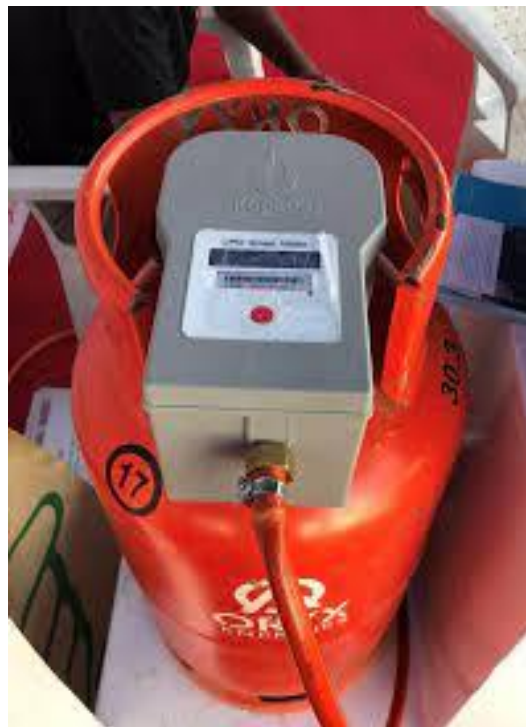
Figure 2-1: Smart meter fixed on LPG cylinder Source: Ndunguru 2019
