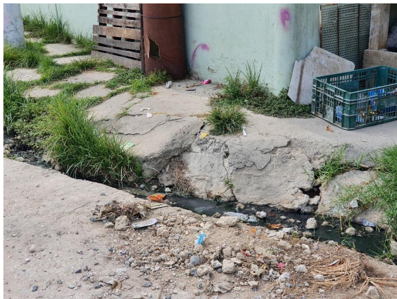
Figure 13: Sewage flowing through an open ditch directly to the storm drain system near Old Point (Photographer: Juan Diego Ayala)
