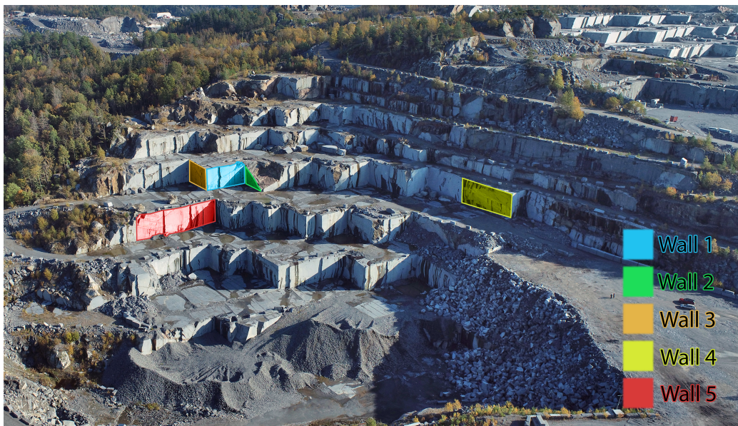
Figure 18: Overview of the quarry and the different walls that got scanned. Wall6 is further east and is not included in this figure.
