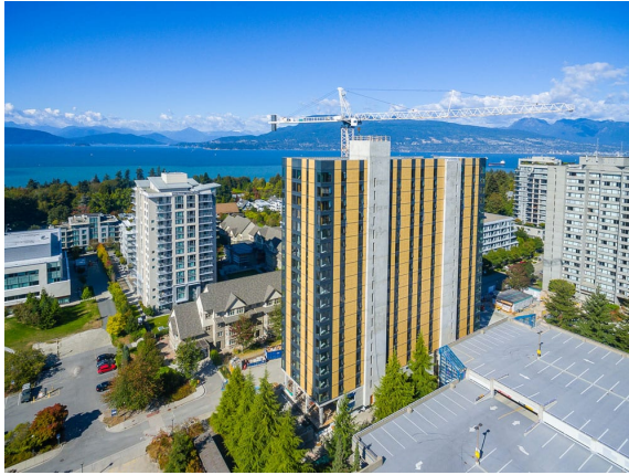
(a) Brock Commons, Vancouver, Canada. Mass timber building with concrete stair core (Think Wood, 2020).
