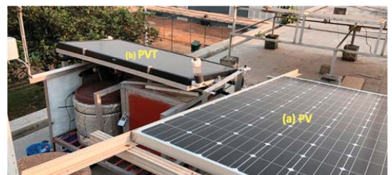
Fig. 1. PV (a) and PVT (b) setup on the rooftop of the Solar Energy Applications Laboratory at Department of Mechanical Engineering, KNUST Ghana (Abdul-Ganiyu et al., 2020).
