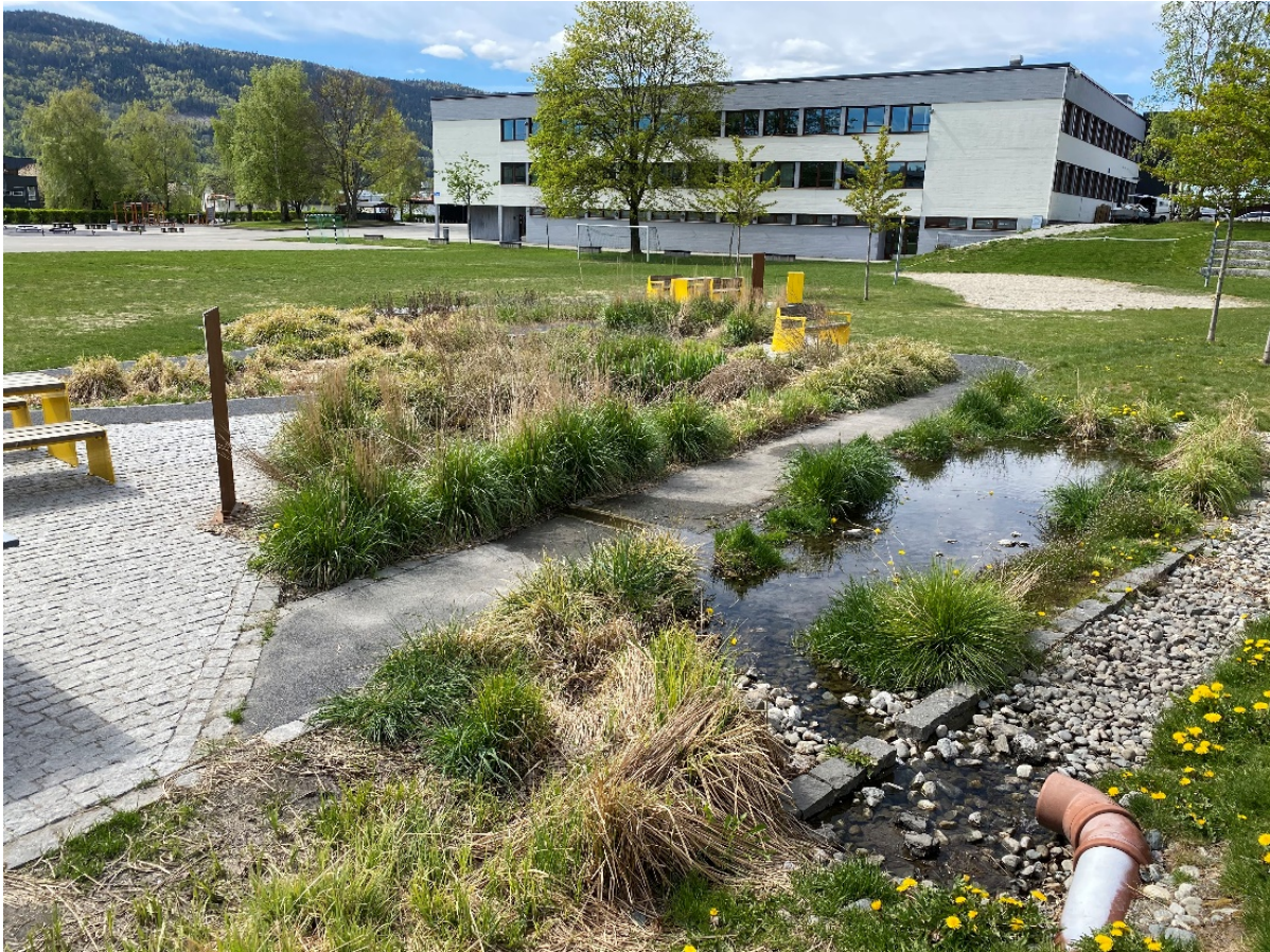
Figure 2.2.1-1: Rain-garden in Drammen municipality for retention of water. Photo: Line Rosef
