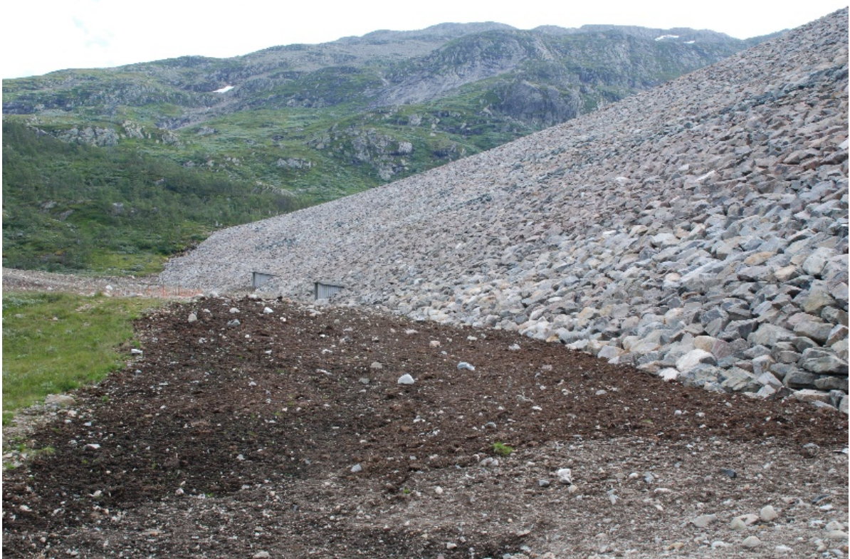
Figure 2.1.5-1: Restoration of landscape and vegetation after hydroelectric power dam rehabilitation approx. 950 m.a.s.l., Bitdalen dam, Vinje municipality, Vestfold and Telemark County. Photo: Line Rosef
