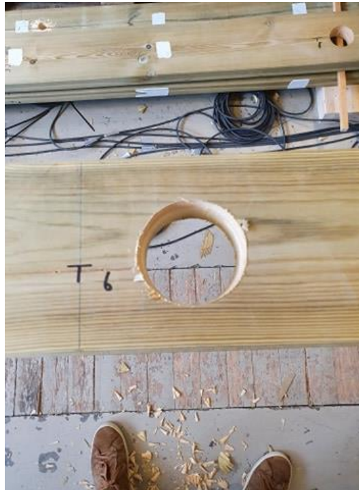
Figure 4.53 - Hole at mid-point of beam
