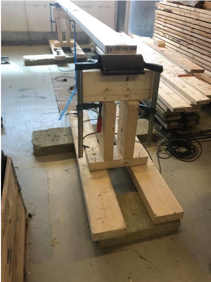
Figure 4.46 - Simply supported beam on steel rollers with insulation beneath support
