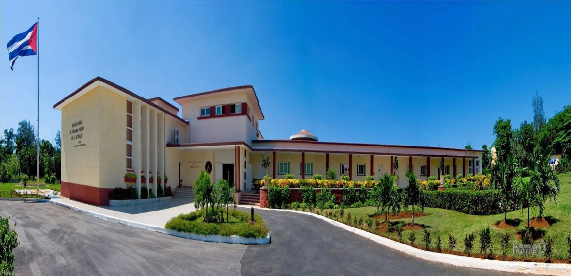
Figure 2-1: Cuban National Civil Defence Headquarters (EMNDC) (Source: EMNDC).
