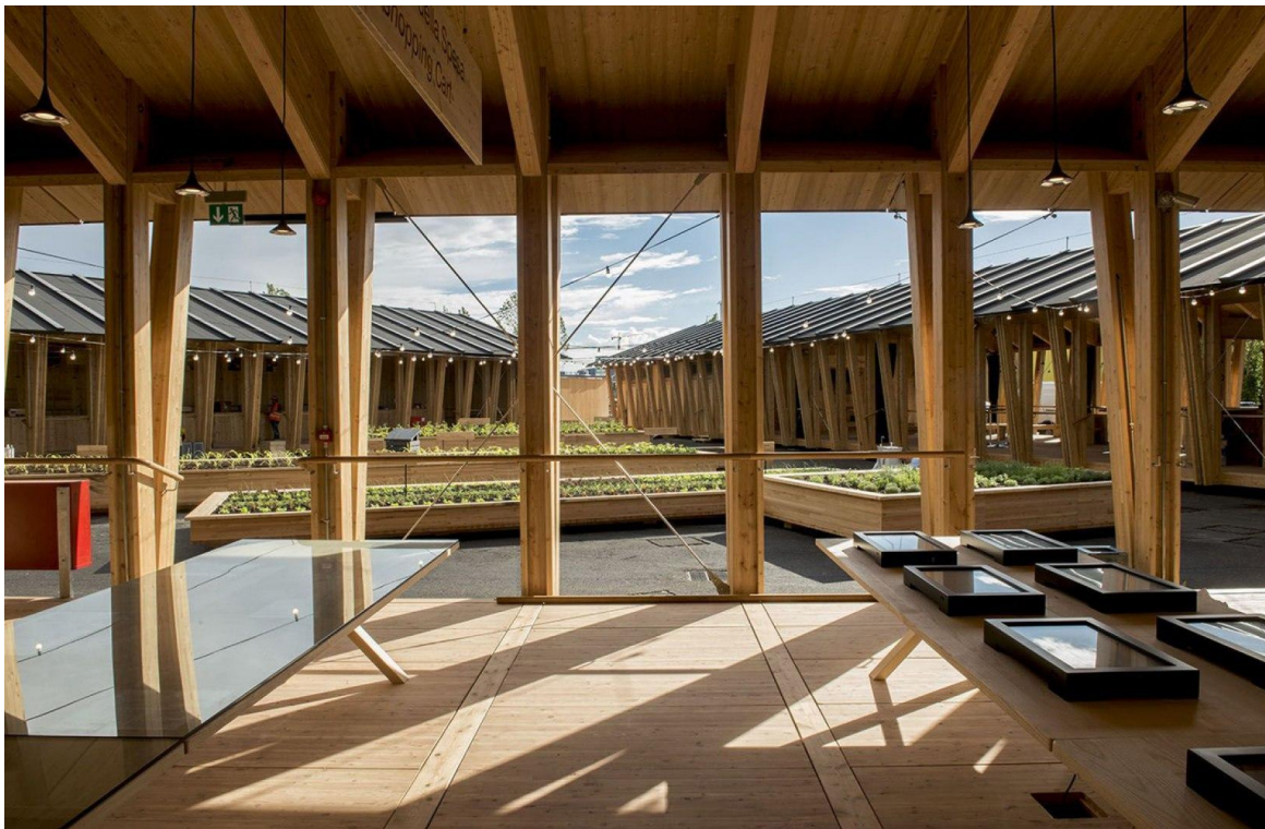
(top) Slow Food Pavilion by Herzog & de Meuron (2015) Photo by Expo Milan 2015 distributed under a CC-BY 2.0 license. Retrieved from: https://www.metalocus.es/en/news/slow-food-pavilion-herzog-and-de-meuron
