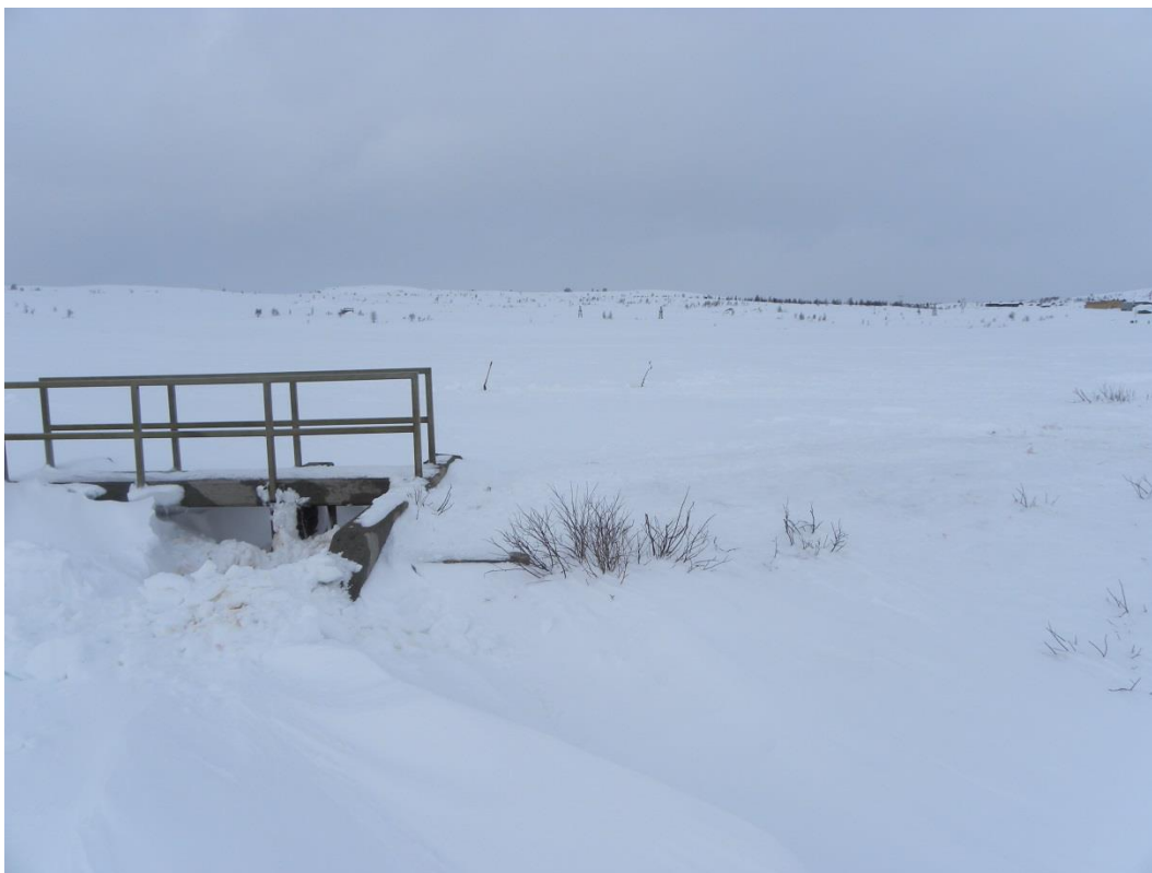
Figure 6: The tailings pond at Storwartz (Pilot) located 9 km north east of Røros, where AMD water for the pilot studies were gathered.
