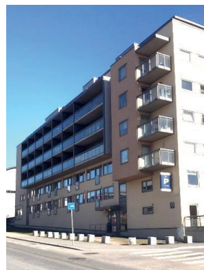
Figure 35. Case project in Gladengveien 15; (photo source: author's own photo).
