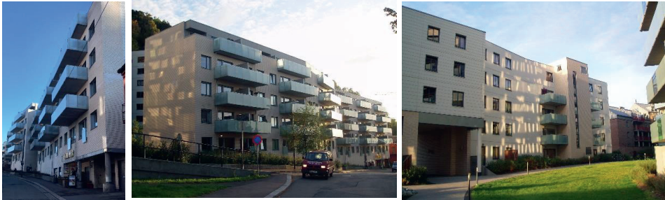
Figure 50. Views of the case in Ekebergveien 5 A–E; source: author's own photos
