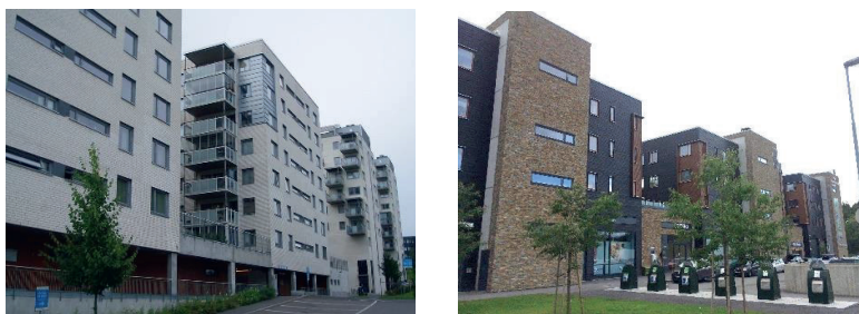
Figure 44. Examples of the main podium type (with the lowest storey above the street-level); location of cases: Grenseveien 50–58 (left) and Helga Vaneks vei 1–3 (right); image sources: author’s own photos
