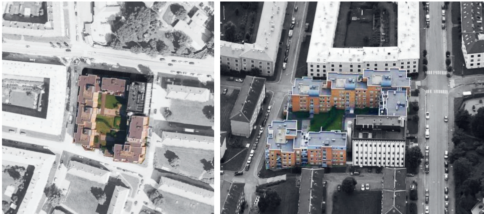
Figure 13-7 Inner courtyard infill – Schouskvartalet (completed in 2009); Photo left: © Oslo kommune, Plan- og bygningssetaten. Rendered with permission of copyright owner. Photo right: © Blom.
