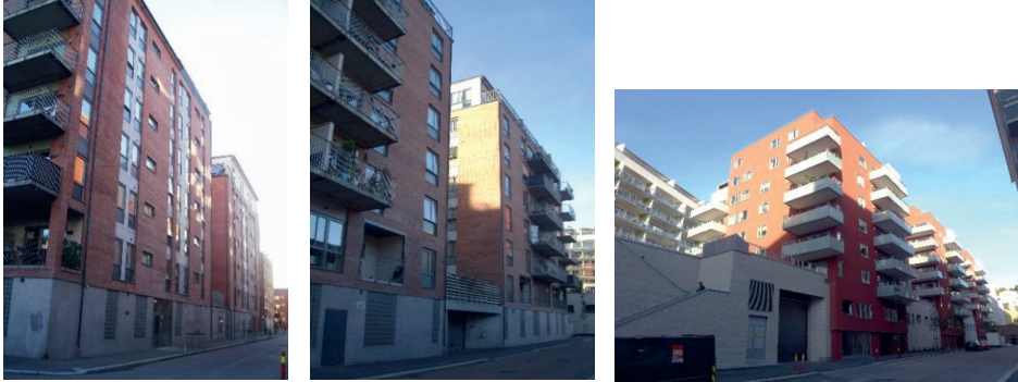
Figure 51. Blind street-level that podium type occasionally creates; case projects located in Turbinveien 9–13 (left and middle) and Turbinveien 4B–24 (right); image source: author’s own photos
