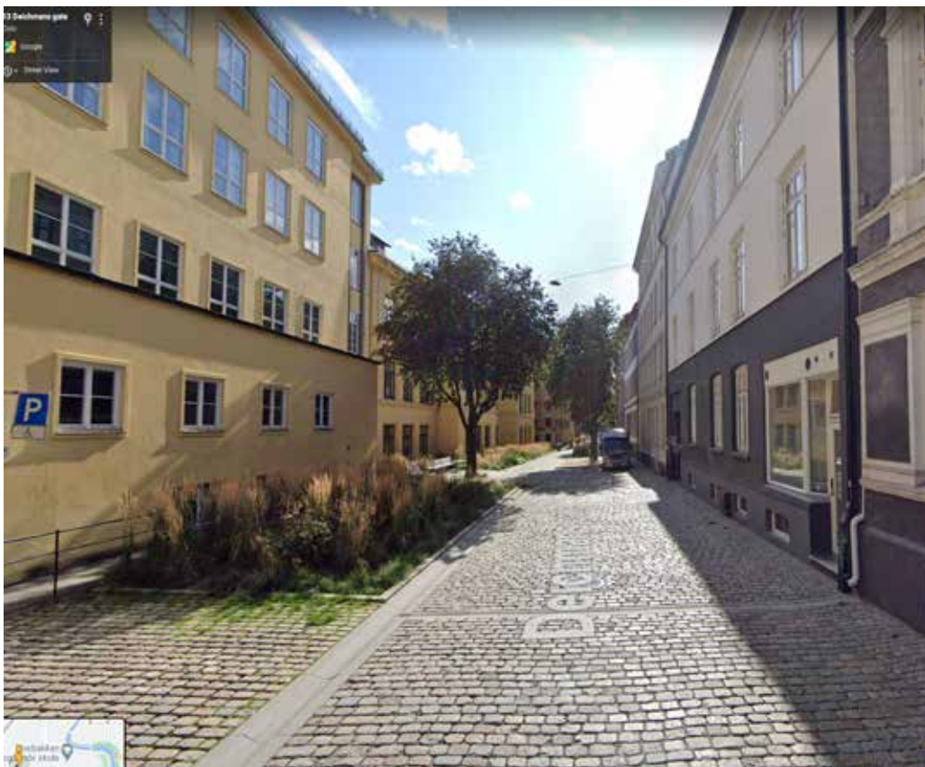
Photo. 5.32 After: surface water from the roof on the right is led to a gutter which feeds in to the rain garden (?) on the left.
