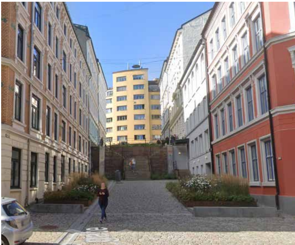
Photo. 5.34 After: Three trees have been removed and replaced with tiered rain gardens and stone sculptures.
