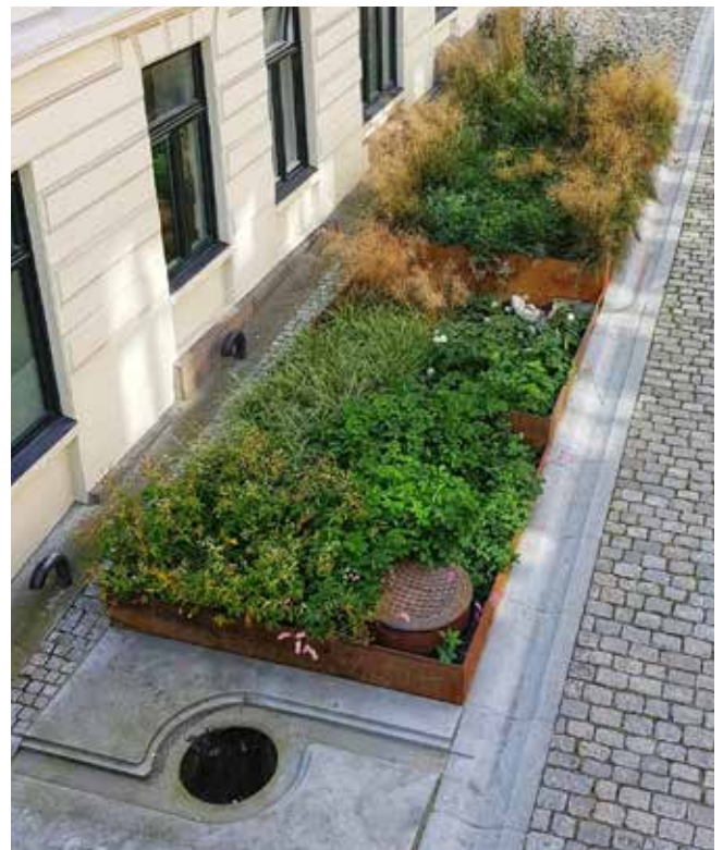
Photo 6.6 Testing in the lower two sections of the planted area. JRE
