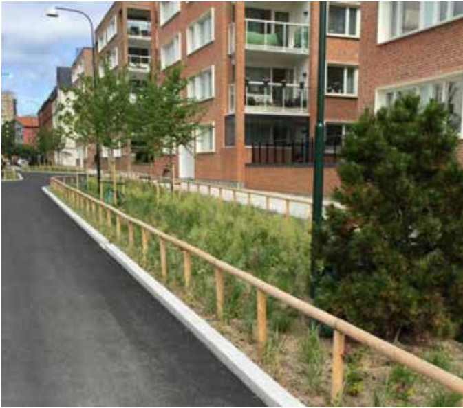
Photo 4.1 The use of rain gardens, for instance in Monbijou street, work to gather stormwater and create a better traffic environment (ibid, p. 36).
