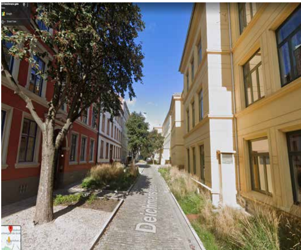
Photo. 5.28 After: the existing green structures have been extended and converted to rain gardens, while remaining surface areas have been made permeable through the use of gravel and cobblestones.
