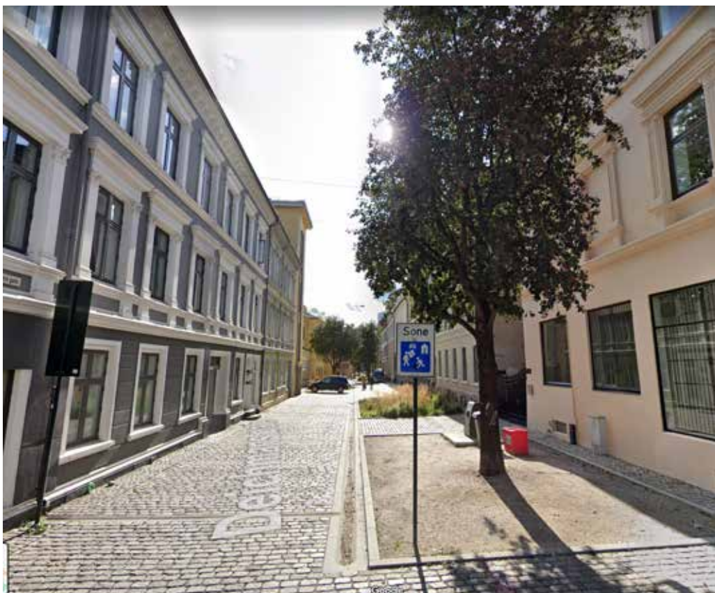
Photo. 5.30 After: Rain garden 7(?) visible on the right side of the street. Also visible is one of several granite gutters leading to the rain gardens.
