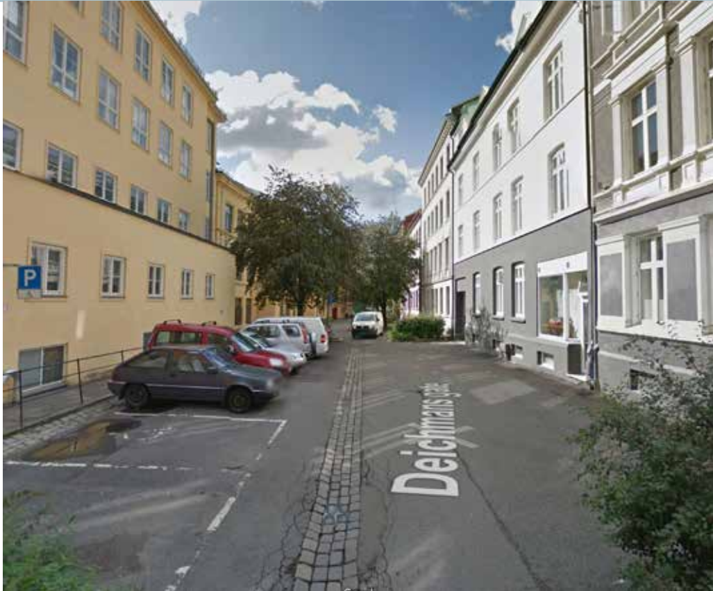
Photo. 5.31 Before: looking south with Møllergata school on the left. Visible standing water in the parking space in the left-hand corner and a clear low point along the middle of the street.
