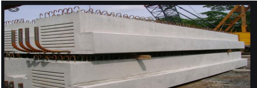
Figure 2-2 it is an example of the reinforced concrete beam precast RC (source by my camera from work site)
