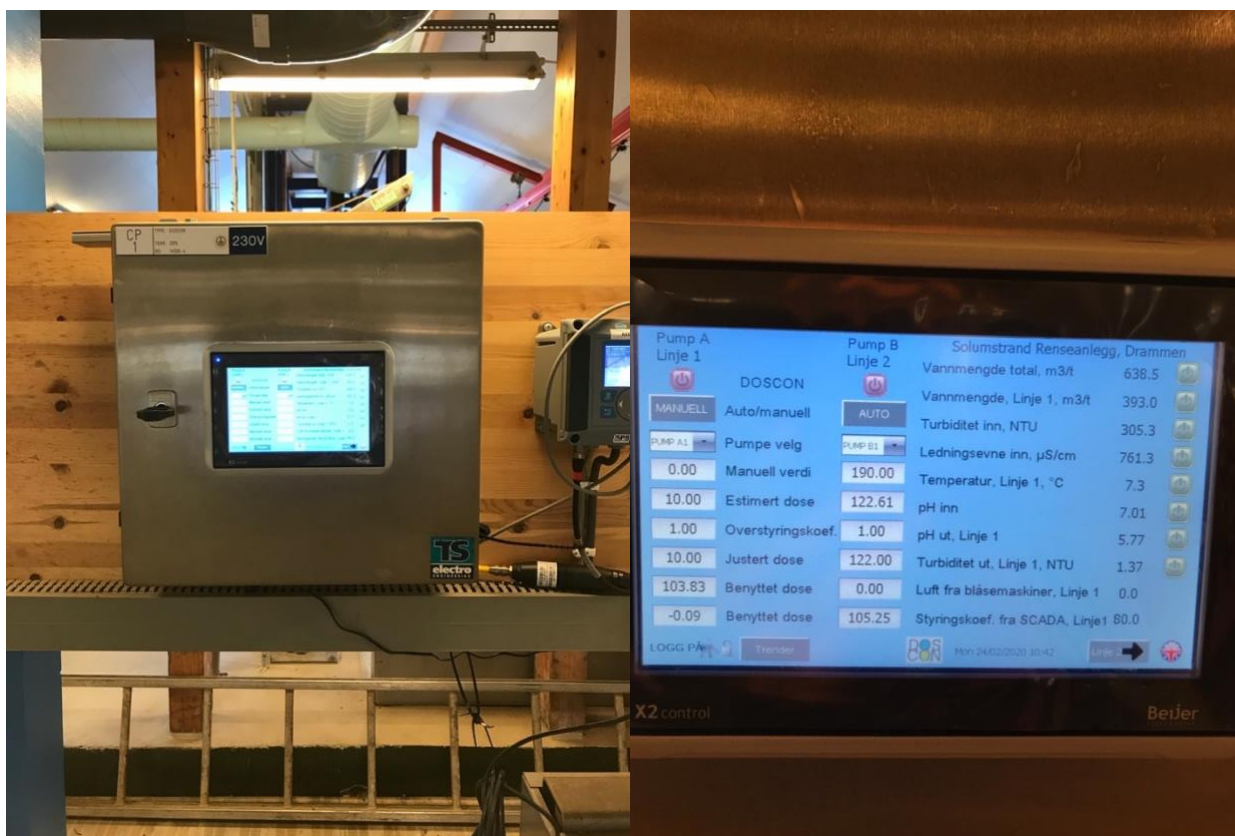
Figure 3-2: The DosCon® controller and the parameters measured by DosCon
