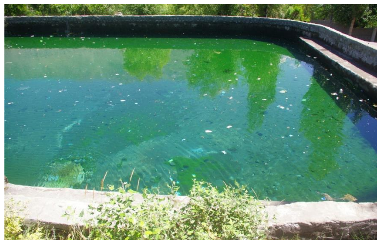
Figure 23 Water Tank Contaminated with Solid Waste Materials
