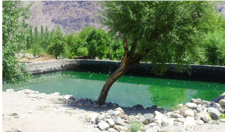
Figure 22 Water Tank for Drinking Water Supply
