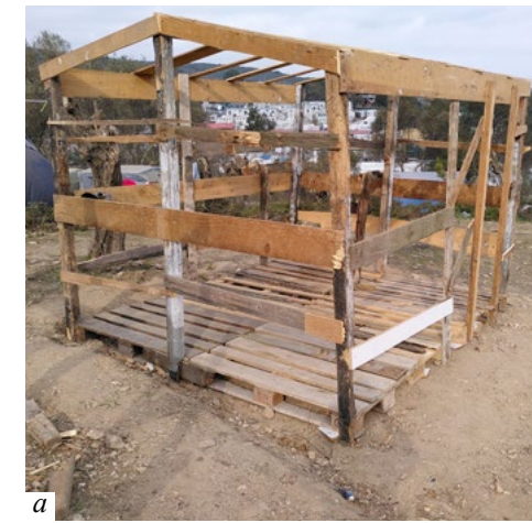
Figure 33. The building and selling of tents creates a property market made by and for refugees. a-c - The construction of a pallet tent, including shaping the terrain, can be done in a day or two.
