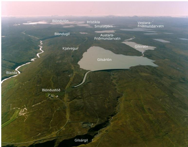
Figure 2 Damsystem seen southwards from Blanda power station. Placenames marked in picture. 2013. Page 12 in LV-2013-117 "Landscape analysis of the effect area of the Blanda power station" by Landsvirkjun. CC BY-NC-ND 2.0.
