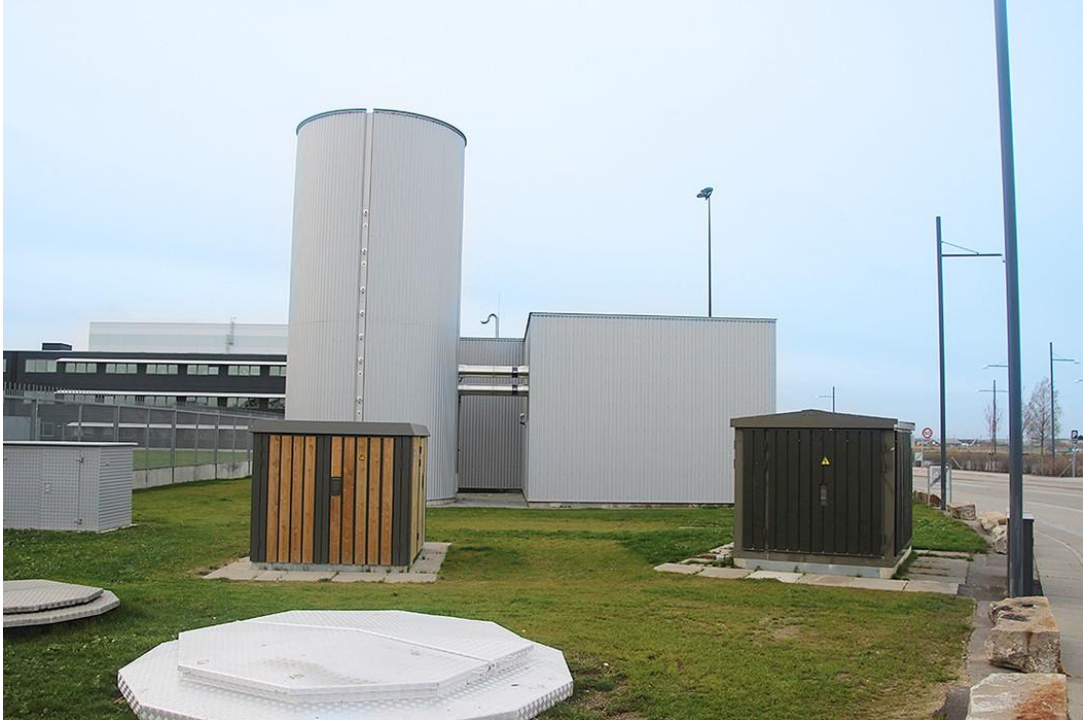
Figure 12: Image showing the FlexHeat virtual battery of 4 MWh stored thermal energy in its 100 m 3 storage tank [60].
