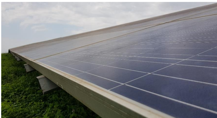
Figure 4.14: In Rwanda I the uniform-distributed dust was a very thin layer of brown/black color, only visible from high angles of incidence.
