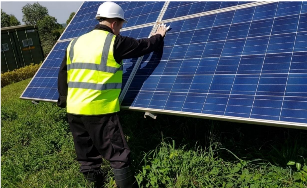
Figure 4.7: Whenever the vacuum cleaner was ineffective (or had broken down), cotton pieces were used for dust collection.
