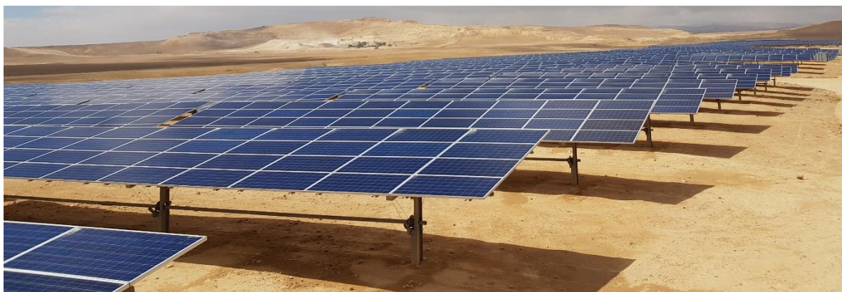
Figure 4.10: The rain in the night between March 16-17 th had cleaned the panels extensively in Jordan II.
