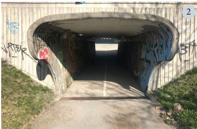
Figur 4.19: Mindre trivelig undergang under Rv282.
