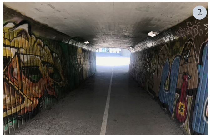
Figur 4.20: Mindre trivelig undergang under Rv282.
