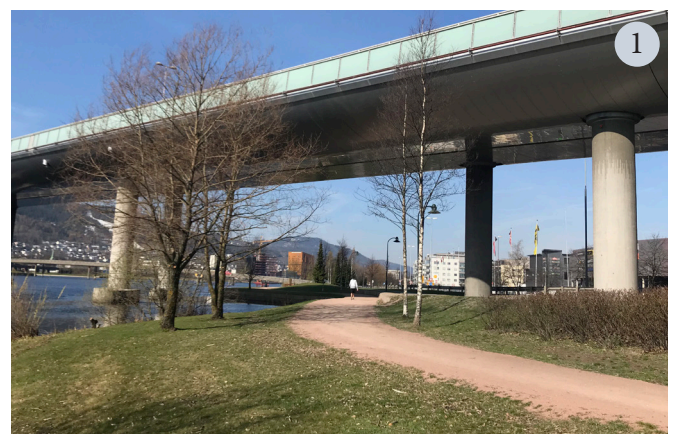
Figur 4.14: Undergang langs elvepromenaden under E18.
