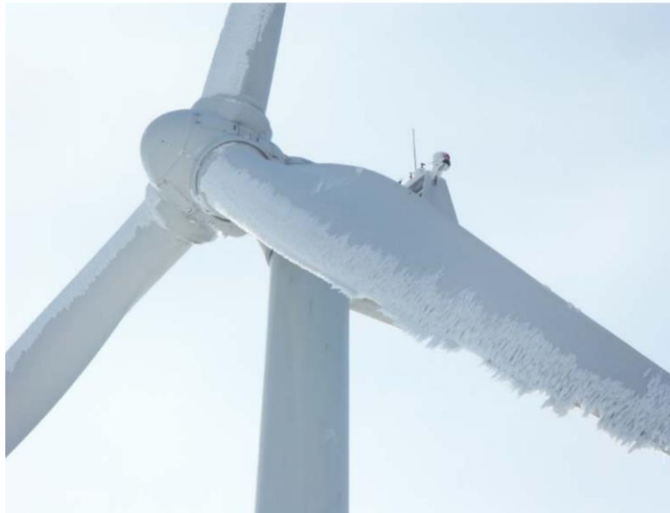
Figure 5: Rime ice on a wind turbine (Ronsten, 2008).
