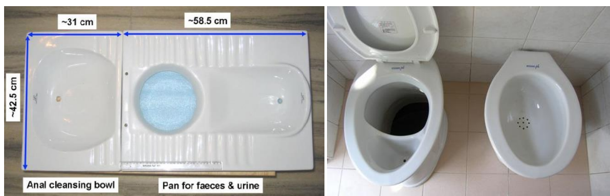
Figure 5.10 (left): Urine diversion squatting pan toilet with a separate anal cleansing bowl (Photo: Johannes Heeb), Figure 5.10 (right): Urine-diverting flush toilet (Photo: Richard Brunt)
