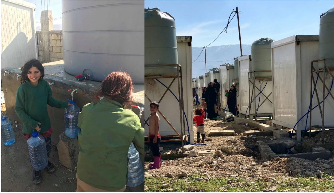
Figure 2.9 (left): Girls that refill their jerry cans in one of the four drinking water tanks in Yasmine camp Figure 2.9 (right): Each household is connected to the pipe network and the pumping line goes to their 1000-liter non-portable storage water tank
