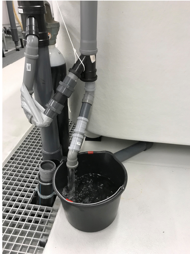
Figure 38 Demonstration of the manual water flow measurements
