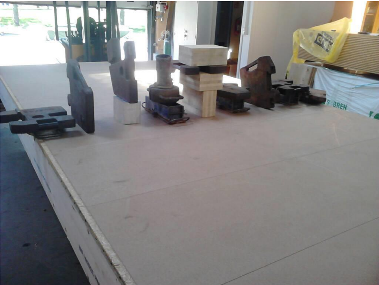
Figure 4.7 - Loading of nine joists
