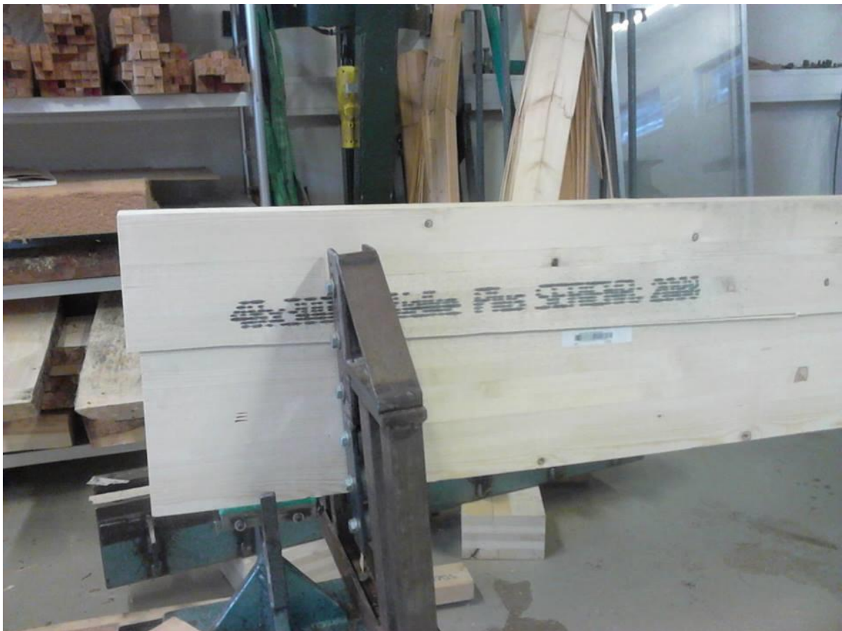
Figure 4.21 - Shear failure of beam
